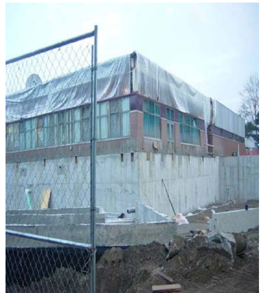
Foundation poured next to building
