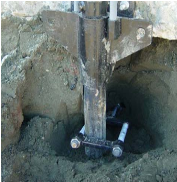
Tie-Backs installed for Lateral Support
